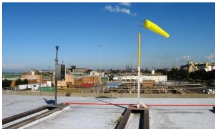
Figure 20: PKCT northern continuous dust monitor
