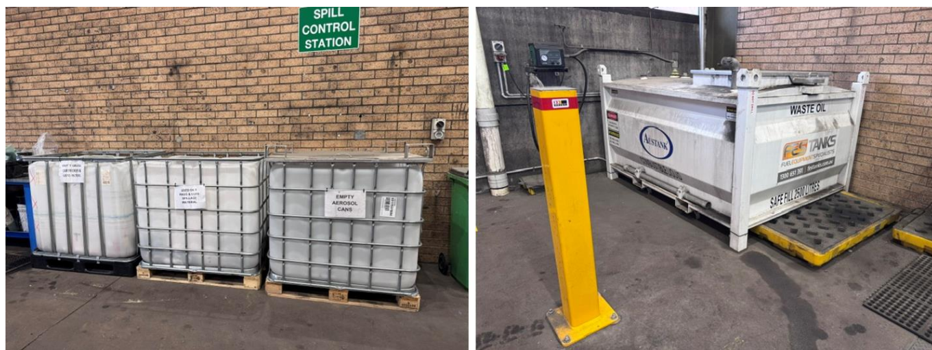
Figure 39: Recycling points for oily rags, aerosol cans, grease cartridges and waste oil
