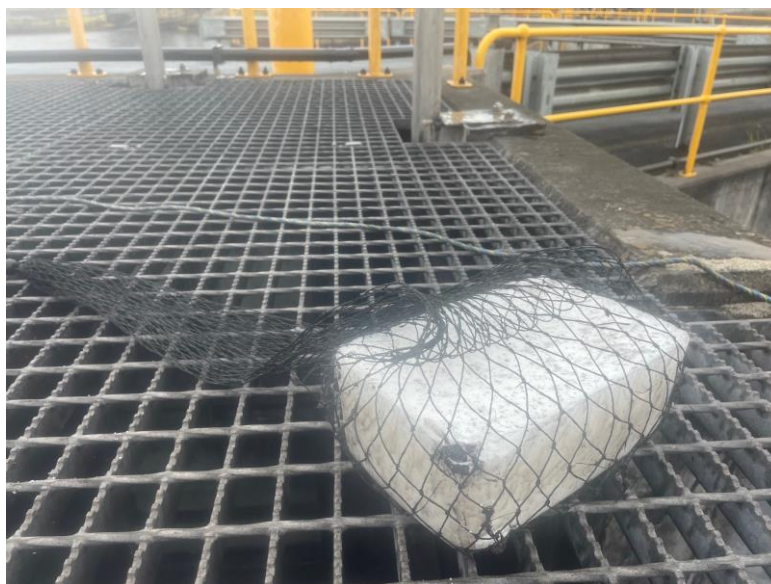
Figure 28: Floc Block in use at Central Pond
