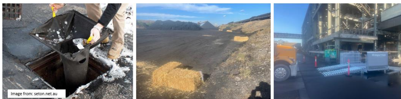
Figure 29: Drain Warden, hay bales and portable truck wash used to manage sediment and contaminant transfer
