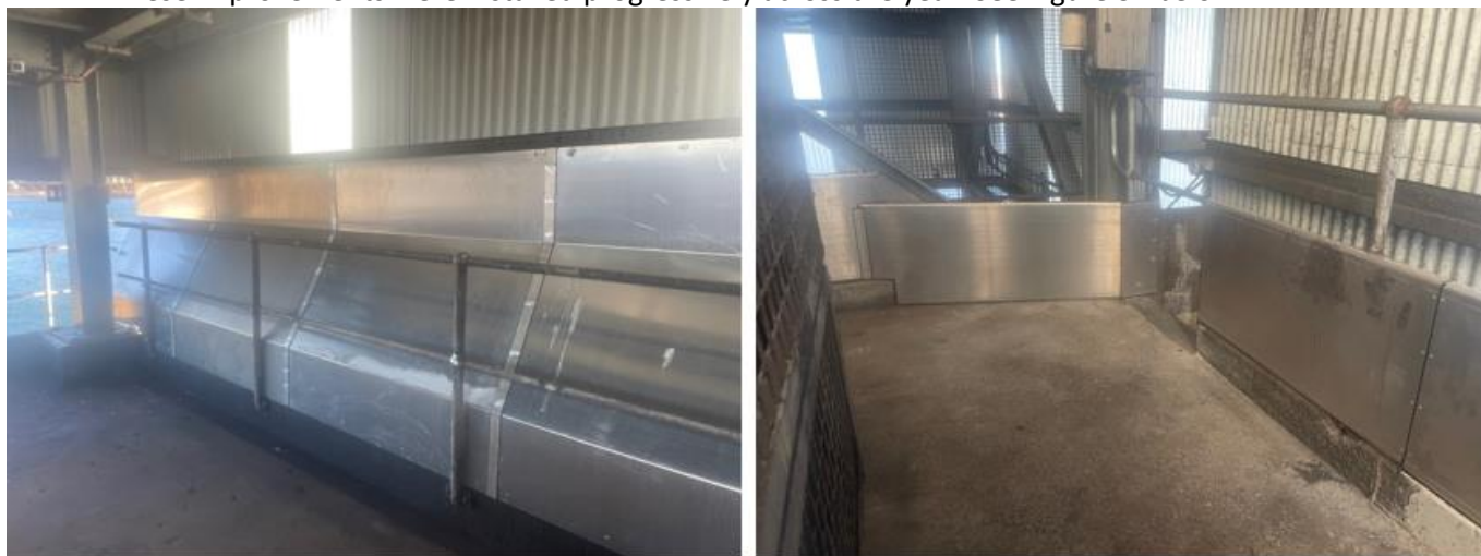
Figure 32: Transfer Station 8 wash down spray deflectors and drainage upgrades
