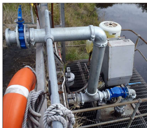
Figure 29: Upgrade to CWCT System – Non-return valves fitted to TS1 and North Pond Pumps.
