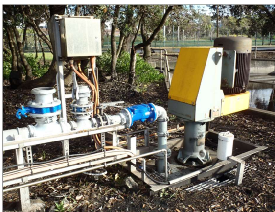
Figure 29: Upgrade to CWCT System – Non-return valves fitted to TS1 and North Pond Pumps.
