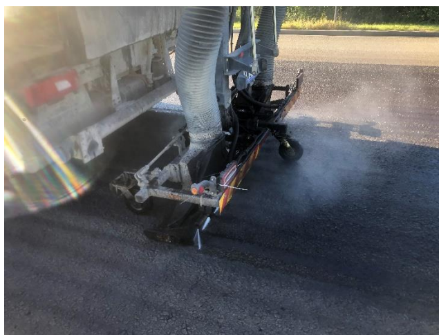
Figure 19: Trial of jet blaster truck to improve washing process of roadways and hardstand areas.
