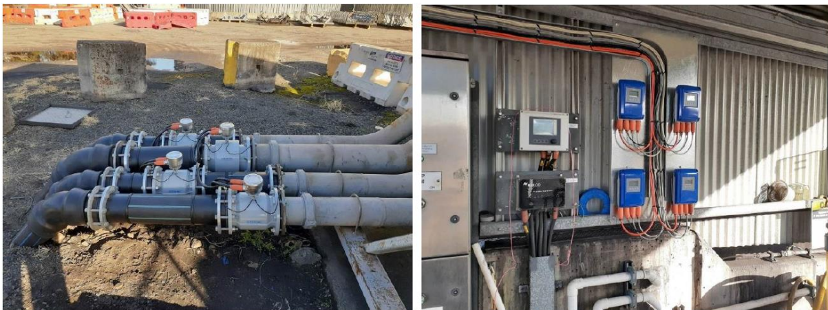
Figure 31: Settlement Lagoon Mag-flow meter installation
