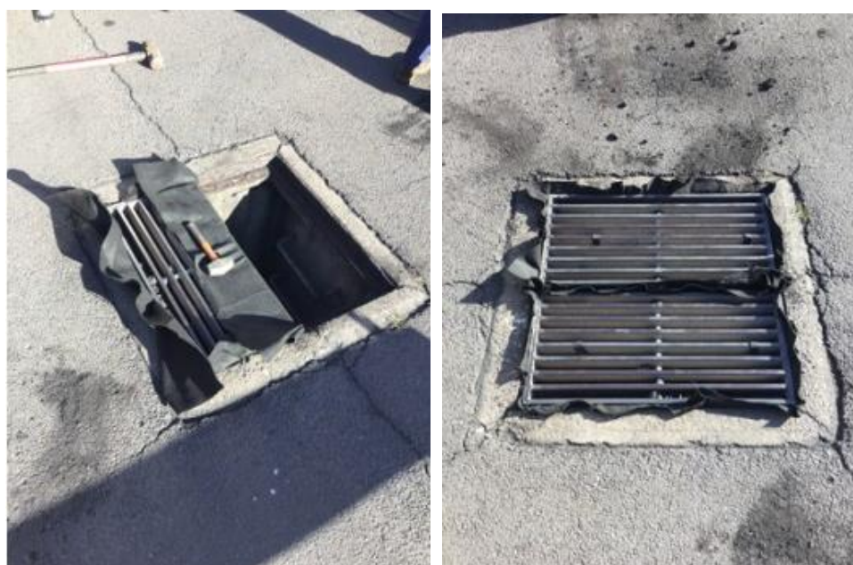
Figure 30 : Install of “Drain Wardens” around Workshop and Store.
